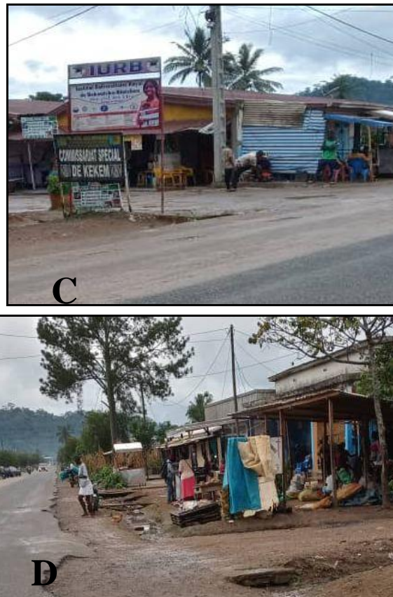
Figure 7. Dilapidated Buildings along the Kekem Transit Area
